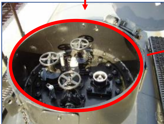
Valving inside the \frac{3}{4} " protective housing
