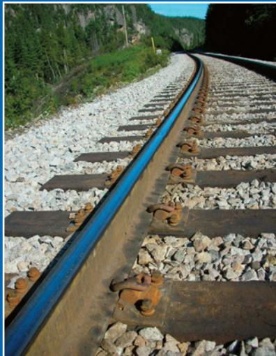
**The Pandrol Victor® system combines the durability of an AREMA tie plate with the benefit of resilient fastenings.**
